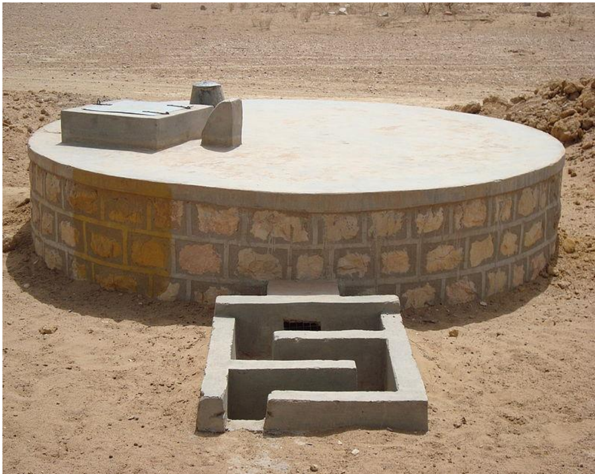
Image 6: Rainwater harvesting tank
